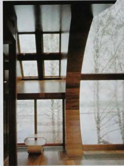
is used for sail storage. The geometry of the building, with its curvilinear surfaces and multiple angles, meant that almost every board composing the inner and outer skin of larch had to be shaped individually. The roof is of copper and the house sits on a reinforced concrete slab.
